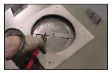
Figure 9.3 Cut the metal retaining band and fold the sides out.
